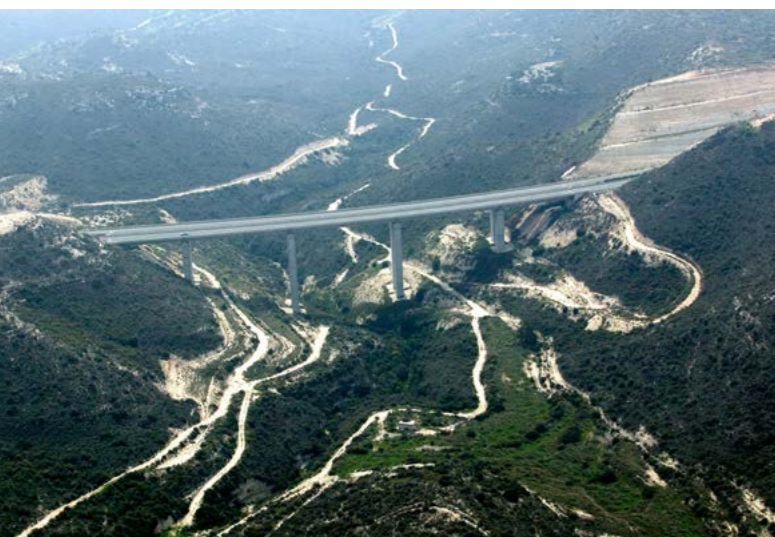
Limassol - Pafos Highway
